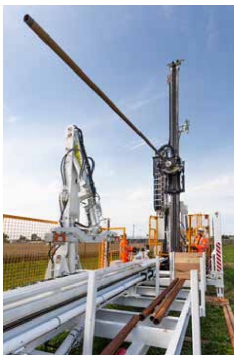
The demand to do the drilling work in a safer way has made the drilling equipment increasingly autonomous.
